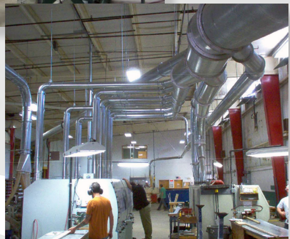
Right: After installation of Nordfab ducting.
