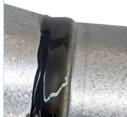
Caulked Seams and Joints on Branches, Elbows, Adapters
