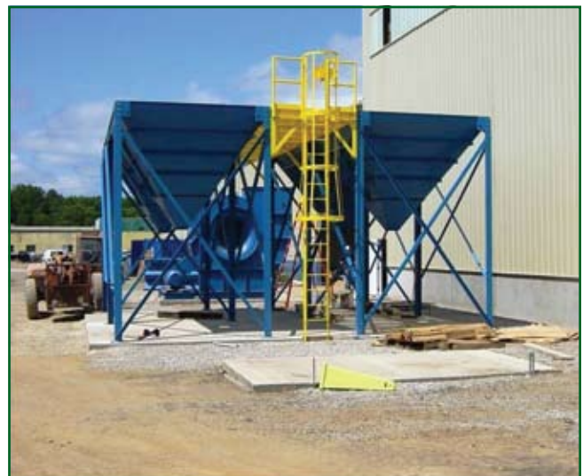
Installing the hoppers.
