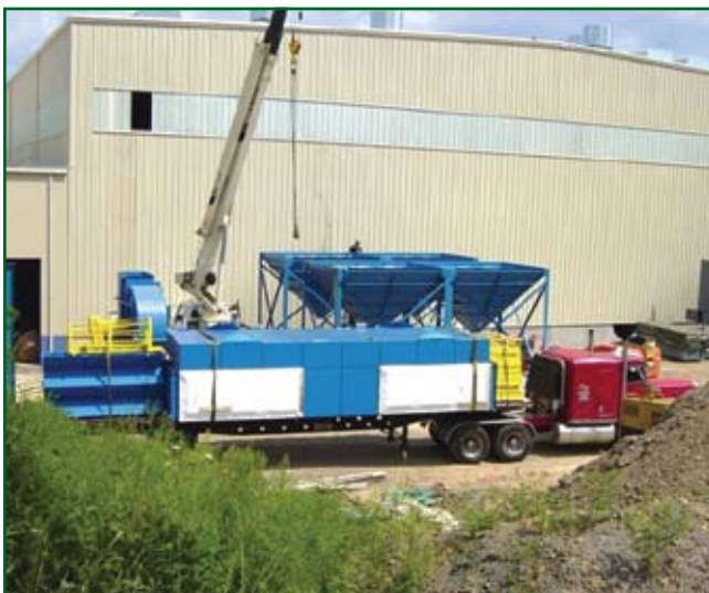
Setting the collector in place.
