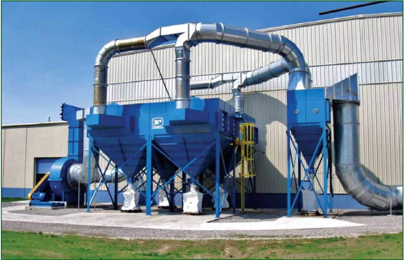
Gold Series model Tandem GS96 collecting fumes from metal processing.
