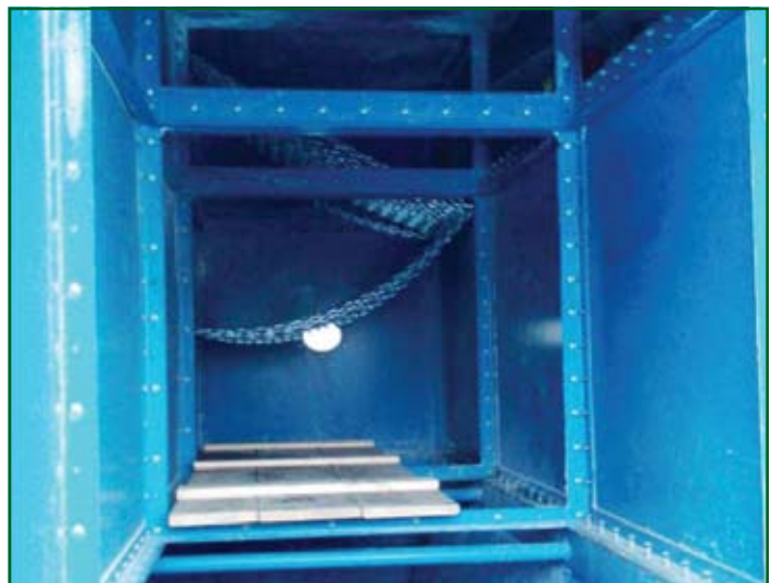
Inserted chains in drop out box.
