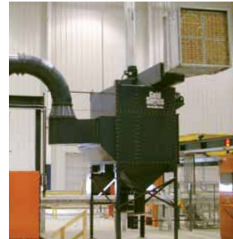
Abrasive resistant inlet, top mount fan, silencer and safety monitoring filter.
