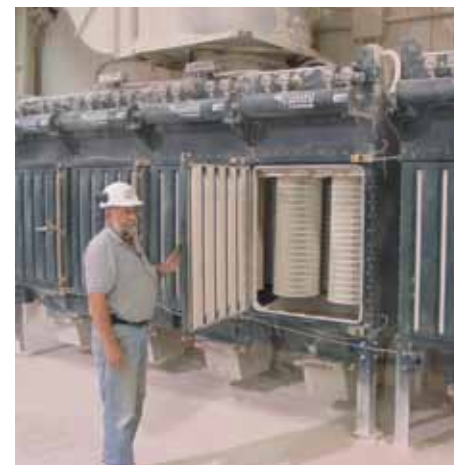
Louvered door inlet for cross-flow applications.
